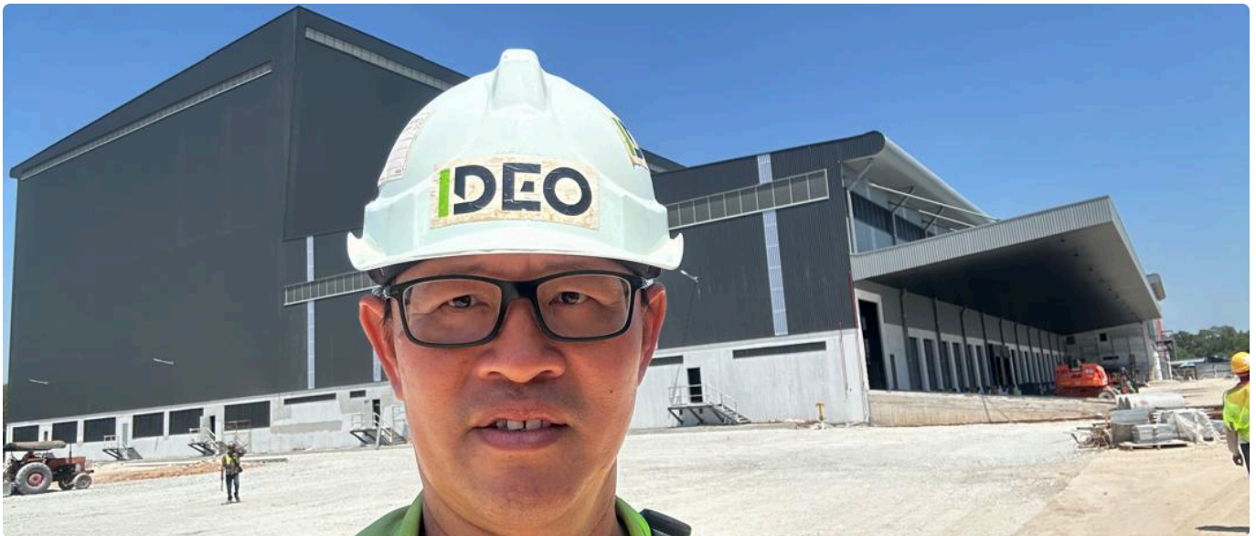
Warehouse nearing completion — external works and hardstanding done
