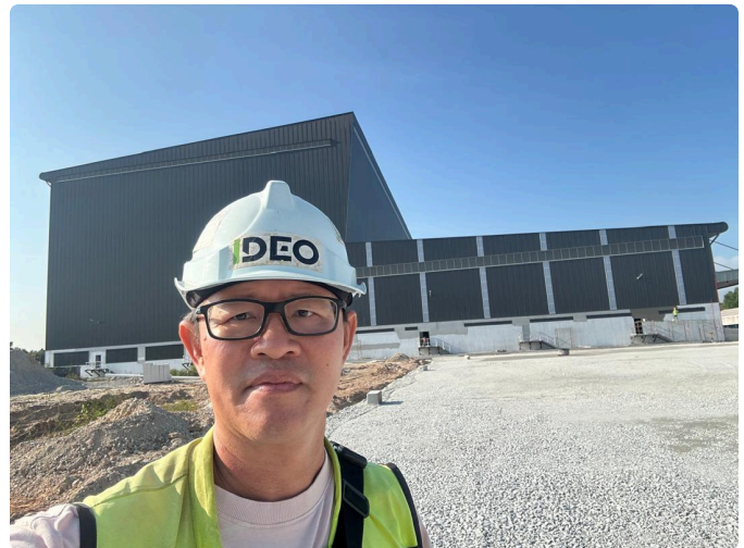
Structural steel and cladding — warehouse completion
