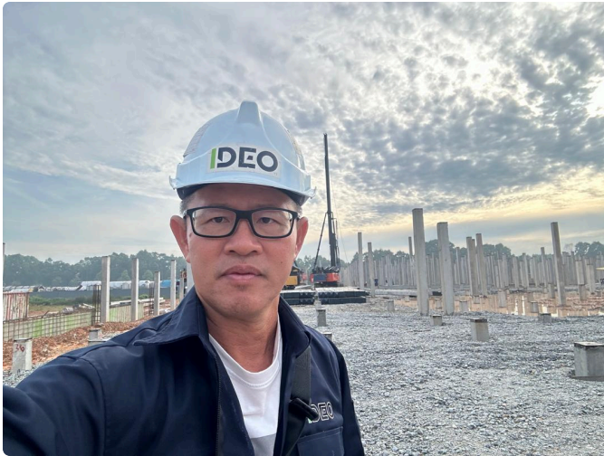
Piling stage — RC Square pile installation work
