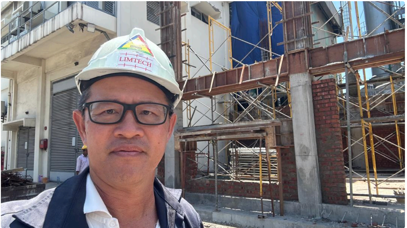
Structural steel and RC works with scaffolding access, adjacent to operating plant
