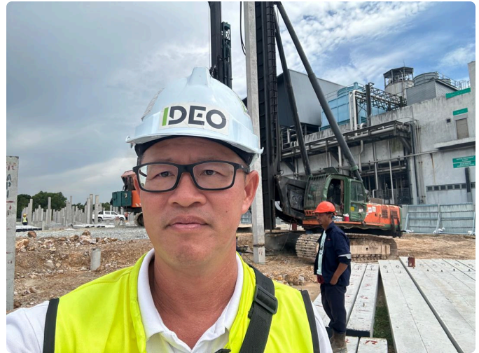
Supervising piling rig operations and pile driving works
